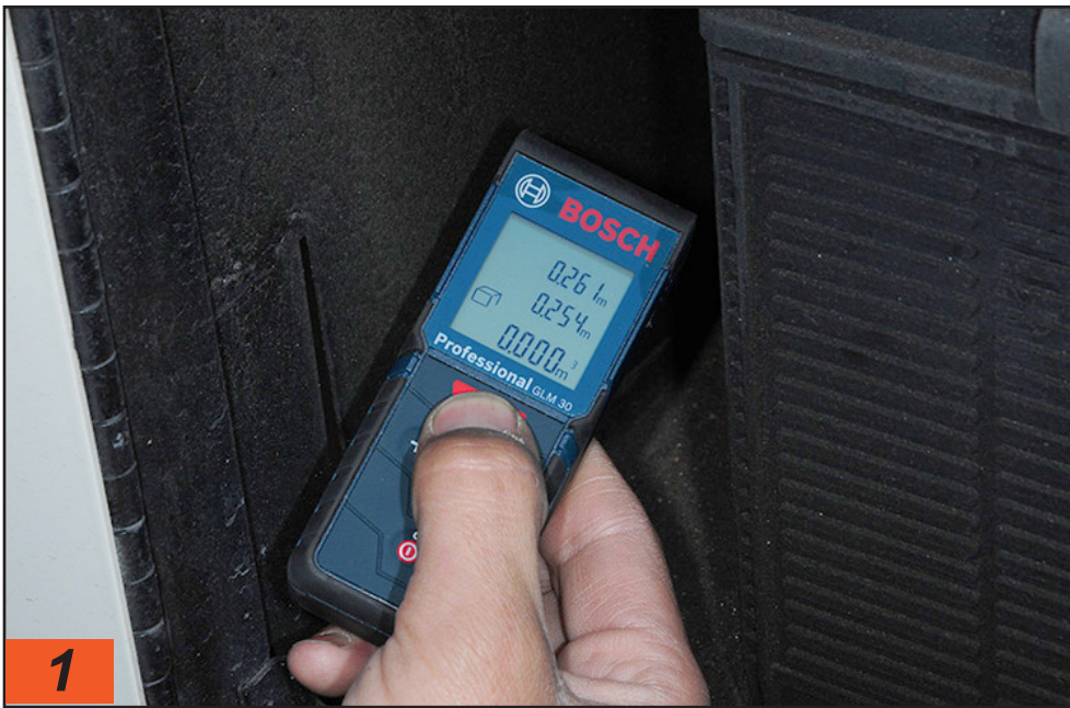
Professional, certified installers start the process by determining the proper device for the area that will be protected. Here the process was started by using a laser measuring tool to determine the compartment dimensions.
