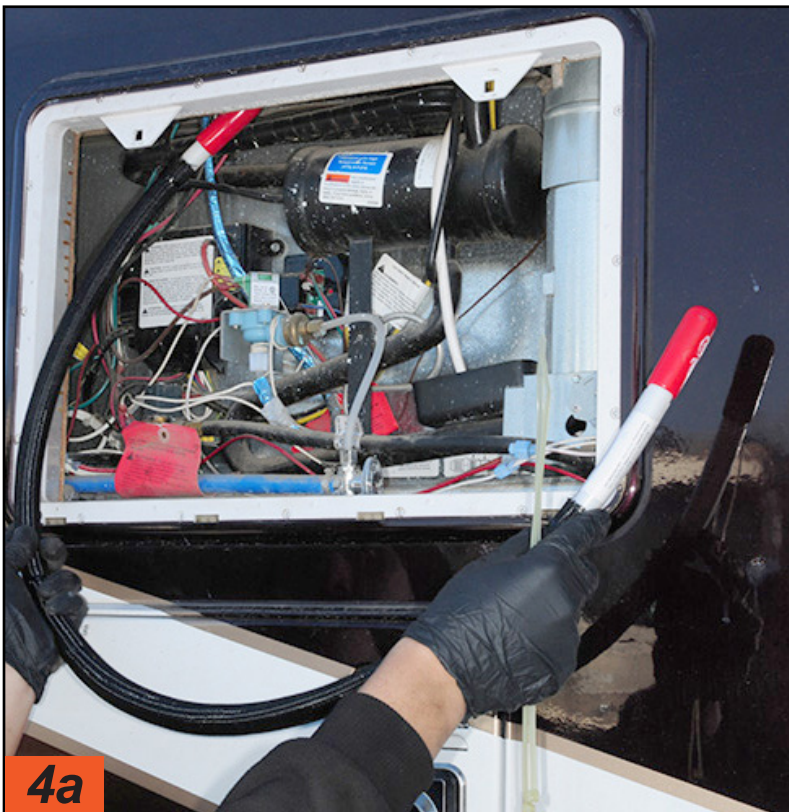
A key area to protect is the back of an absorption refrigerator. Once the device is sized for the specific installation, it's routed from the bottom of the refrigerator, through the bottom access (vent) panel. Care must be taken to clear wires and other components. Since the device is custom manufactured for the exact refrigerator, it will fit nicely in the compartment and terminate in a logical place. From here the device is cable-tied to the back of the refrigerator; for higher heat areas the device is wrapped in a heat shield.
