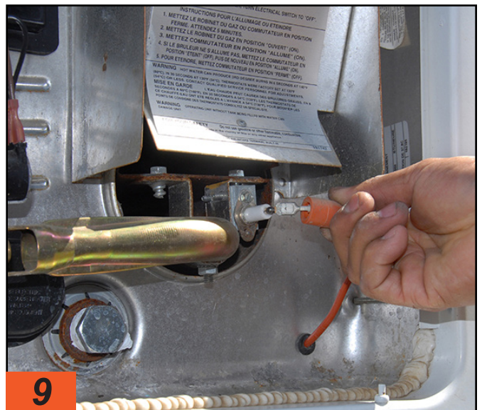
9 Although it looks different, servicing a Suburban water heater is a similar process. First, unplug the electrode wire, as shown.
