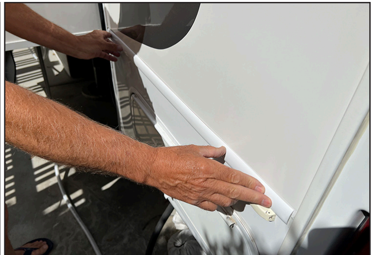
After cleaning the entire length of the sidewall surface with alcohol, the molding was “stuck” to the wall, being very careful to keep the line straight. Finish by running a narrow bead of white silicone along the top and bottom edges of the molding. RVE
