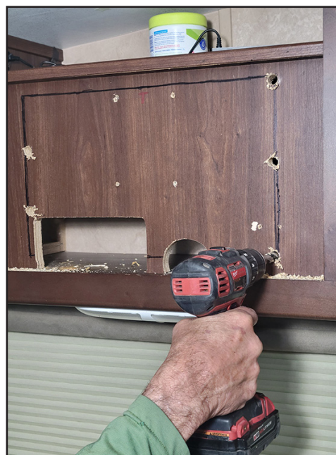
After marking the outline for the cutout, large holes were drilled in several places to make room for the jigsaw blade when cutting in different directions.
