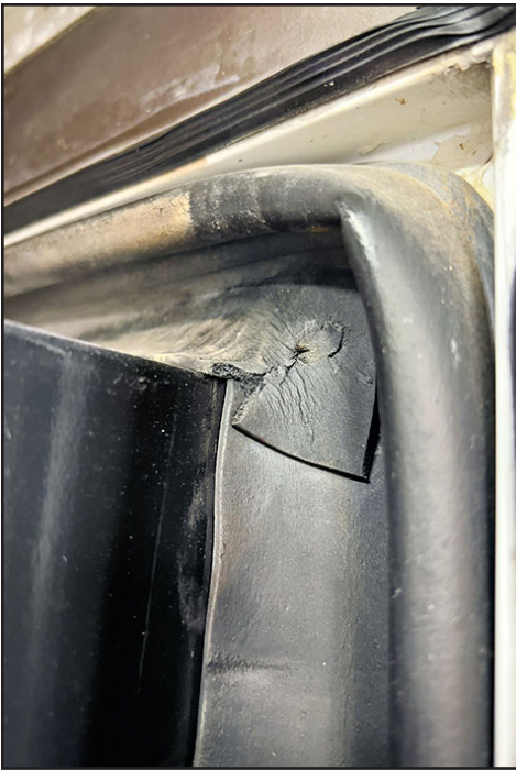
Slideroom wiper seals need to be inspected frequently because they can crack, tear and the corners come unglued, allowing an easy path for water to get inside the RV.
