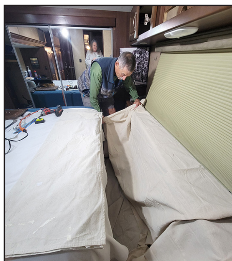
Cutting wood creates lots of sawdust, which was captured by painter's tarps that were spread out over the bed and lower cabinet structure.
