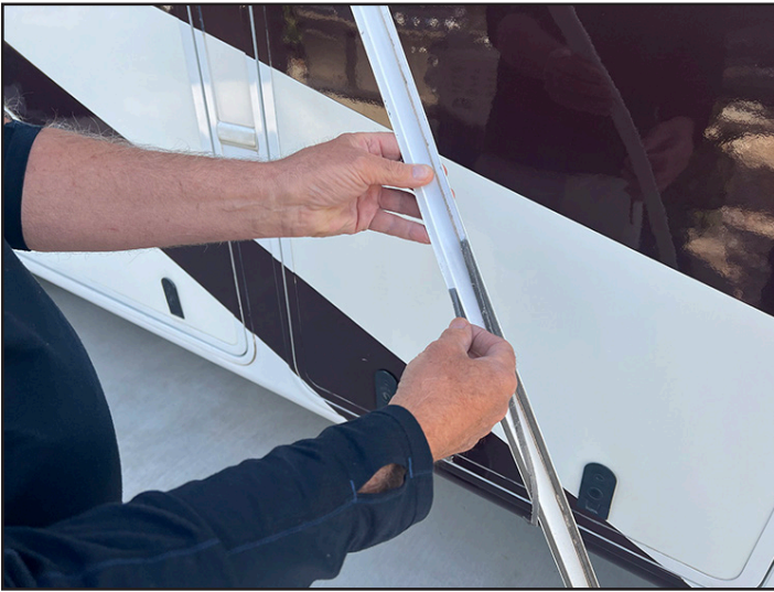
Originally the molding was attached to the sidewalls with foam tape, which actually did a good job for many years. All the remaining tape was removed from the molding before proceeding.
