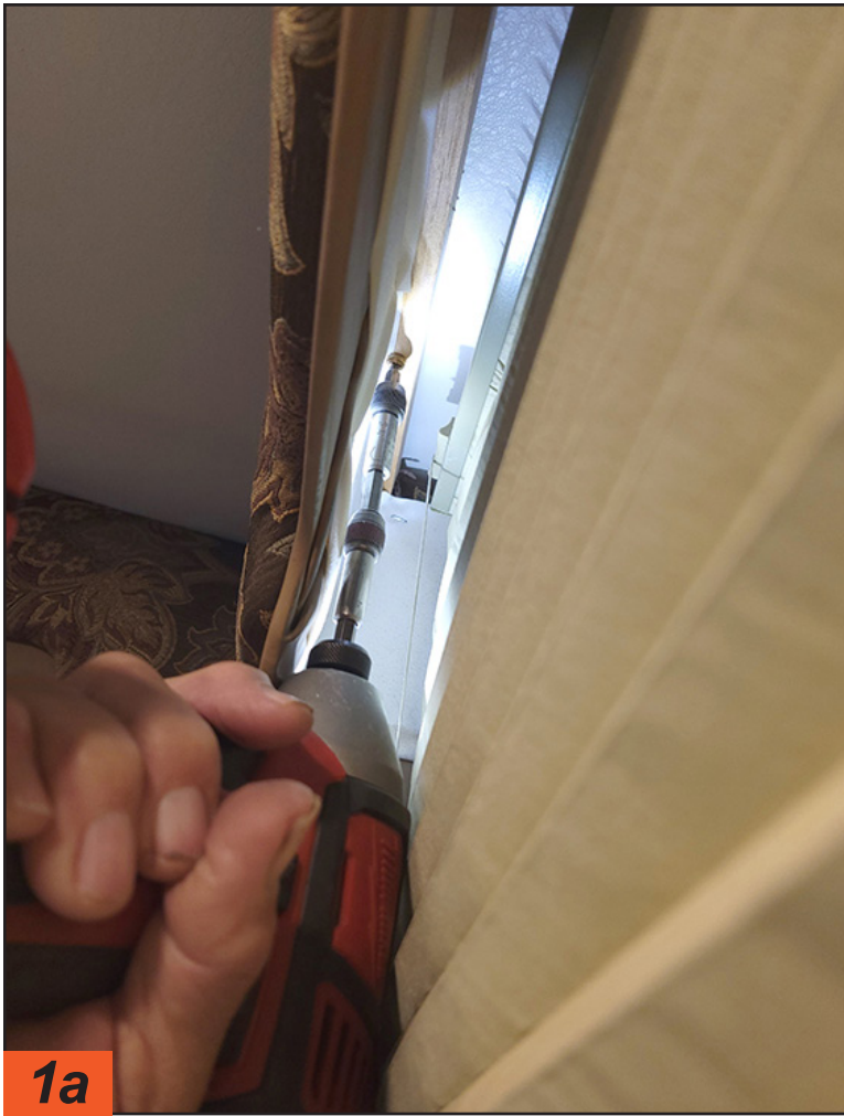
The first step is to remove the valance, which will be slightly different depending on RV model, but most are held in place by a few screws. It's best to use a screw gun or impact driver (on low torque) and a long extension to prevent damaging the valance.
