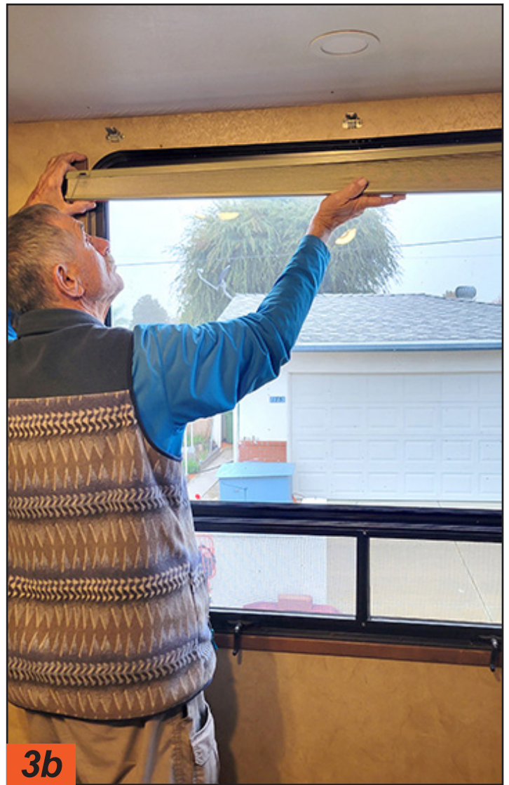
On this Bali Blind it was necessary to use a large, flat-blade screwdriver to release the spring-loaded bracket from the top of the blind. Common day/night shade brackets can be opened by using the screwdriver to twist open the latch. Some of these blinds can be heavy, depending on size, so it may be necessary to recruit some help.
