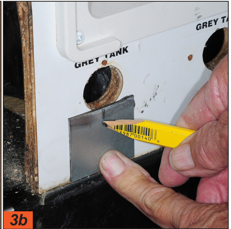
After cleaning the surface with alcohol, galvanized plates were measured and marked for covering the holes, which were way too big for the new cables.
