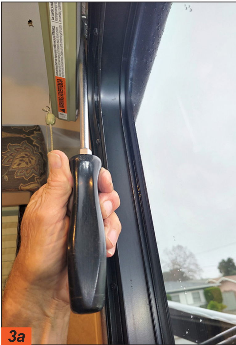
On this Bali Blind it was necessary to use a large, flat-blade screwdriver to release the spring-loaded bracket from the top of the blind. Common day/night shade brackets can be opened by using the screwdriver to twist open the latch. Some of these blinds can be heavy, depending on size, so it may be necessary to recruit some help.
