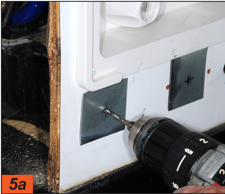
Once the plates were in place, a pilot hole was drilled in the center and then a 5/8-inch hole was cut with a step drill to accommodate the cable assembly.
