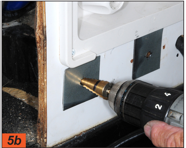
Once the plates were in place, a pilot hole was drilled in the center and then a 5/8-inch hole was cut with a step drill to accommodate the cable assembly.
