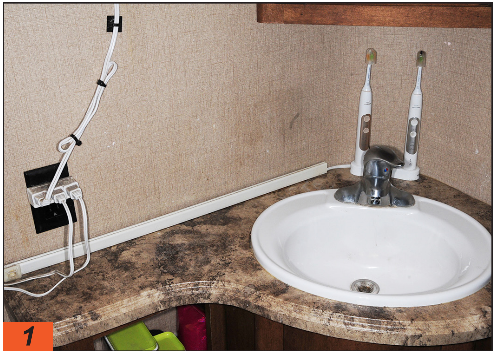
The original routing for the hair dryer and electric toothbrush wiring was an object failure. It made sense at the time, but a fix was certainly in the wings. The biggest problem was the accumulation of dirt on the wire cover that was two-face taped to the wall—and the constant releasing of the double-sided tape.
