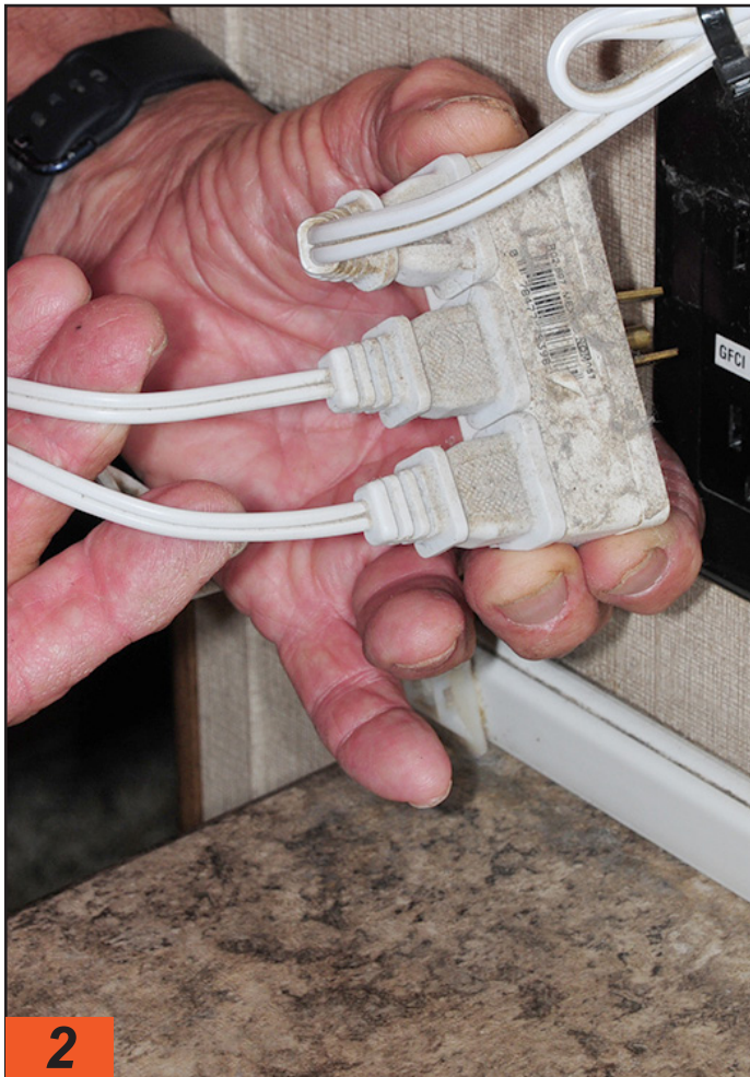
Originally, an adapter was connected to the existing power outlet so the hair dryer and toothbrush could be plugged into 120-volt AC power and leave one receptacle open. It was always a mess — and bulky.
