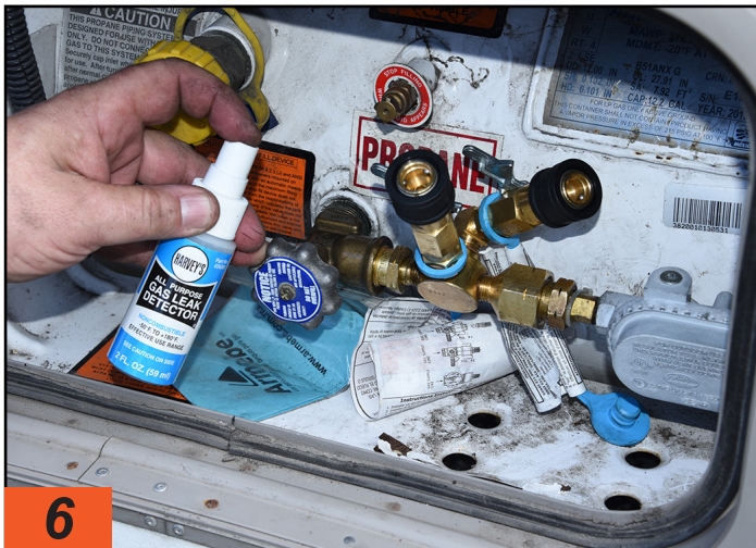
6 Once the fittings are tightened, open the supply valve and spray the fittings with a gas leak detector solution. If there are any leaks, the solution will bubble. You can also use a dish-washing detergent/water solution for this purpose, but do not use Windex glass cleaner or a similar product — the soapy water's surface tension is what allows the bubbles to form and Windex doesn't create the surface tension.
