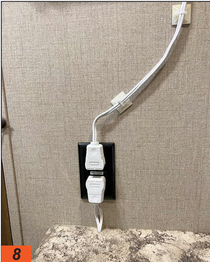
8 Flush-fitting plugs and cable-management tabs keep the wires neatly routed to the power outlet. Hand towels draped over the bar above the outlet (not shown) conceal the wiring for the most part.
