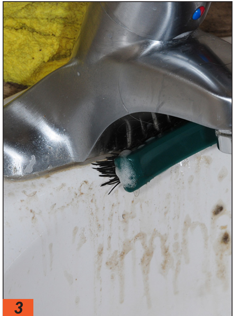
Once the wire covers were removed from the wall, the area was cleaned thoroughly and any corrosion around the faucet base was neutralized with Lime-A-Way and a nylon brush.
