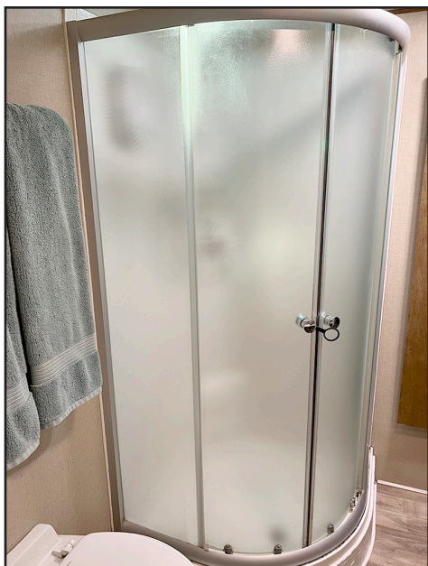
The original garden-type shower stall was stylish, but under the mounting track lurked dirt and grime, which was hard to clean. Over time, the doors were hard to slide open because of the corrosion that built up on the wheels.
