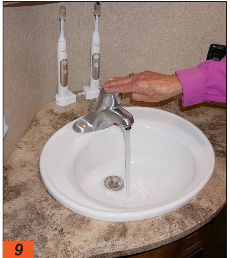
9 Cleaning up the wiring made a big difference in space utilization and cleanliness. The Moen faucet (DF-NML210 SN-RV; $70.90 on Amazon) is a direct replacement designed specifically for RVs. The single-handle mixer allows better control of water temperature. RVE
