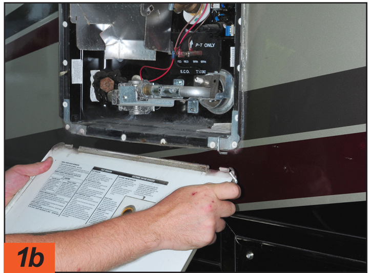
1a The original hot water tank in this motorhome was in good shape, but the owners were full-timers and wanted the convenience of on-demand hot water. The door was removed from the original water heater to begin the process releasing the housing from the side-wall.
