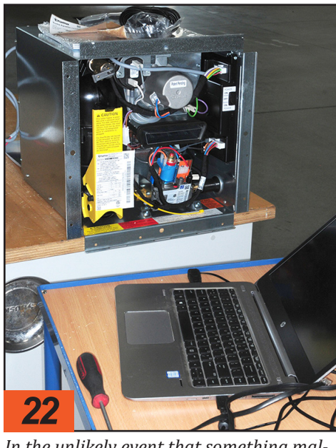
22 In the unlikely event that something malfunctions, the components can be scanned after plugging in a computer with proprietary diagnostic software. All the parts have bar codes specific to respective water heaters.
