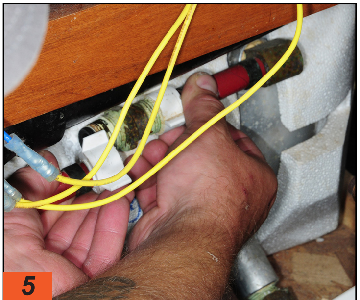
5 All water lines in the back of the old water heater were disconnected before pulling it out of the opening in the wall—of course, after all water sources were closed.
