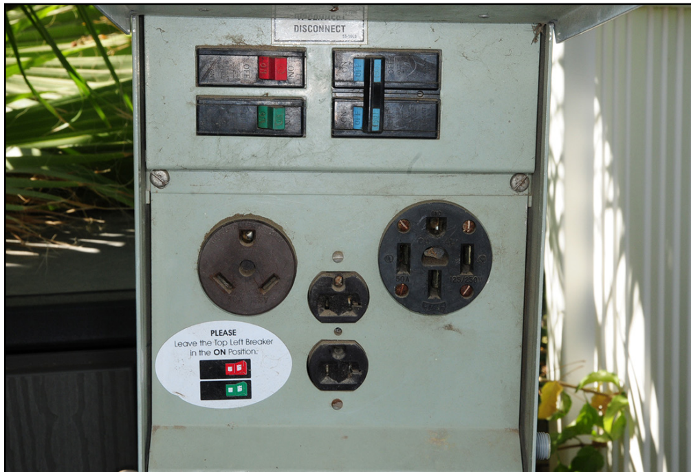
Modern electrical pedestals at RV parks are often equipped with 50-, 30- and 20-amp outlets. A multimeter can be used to check voltage before plugging in the power cord. To test voltage in a 50-amp outlet (shown) put the probes in the common (bottom slot) and one of the two power slots (left or right); the top slot is ground.
