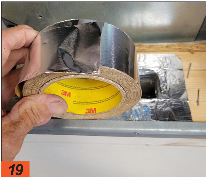
19 It's best to use HVAC tape made by 3M. This is a high-quality tape necessary to hold up in this type of environment for many years.
