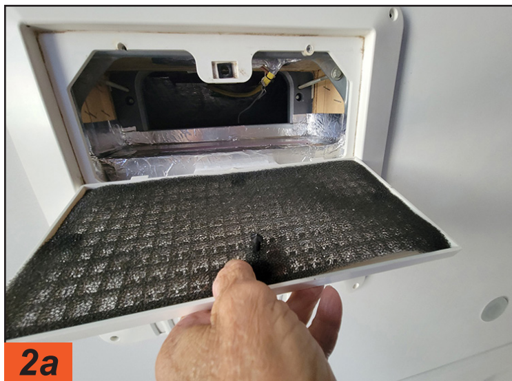
Remove the filter from the return-air access panel so it can be washed with soap and water in the sink. It must be dry before reinstalling and operating the air-conditioner to eliminate moisture gathering in the evaporator.
