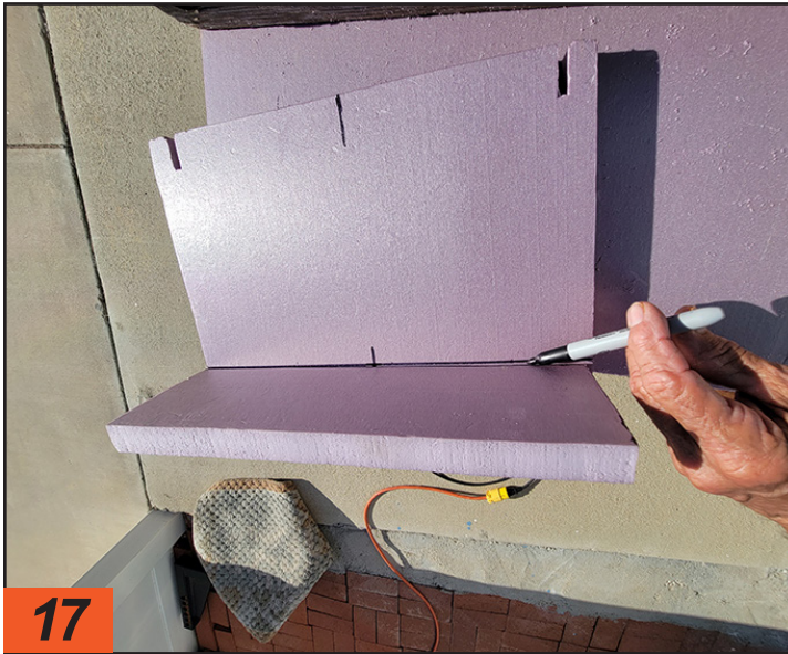
17 The bottom plate is marked at the point where the vertical plate will fit. This step is important because the line will delineate the position of the bottom wedge assembly.
