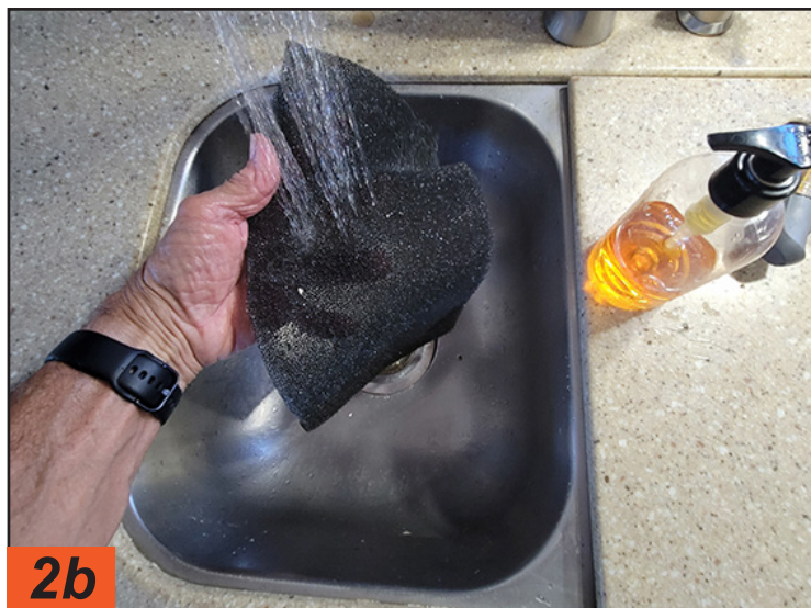
Remove the filter from the return-air access panel so it can be washed with soap and water in the sink. It must be dry before reinstalling and operating the air-conditioner to eliminate moisture gathering in the evaporator.
