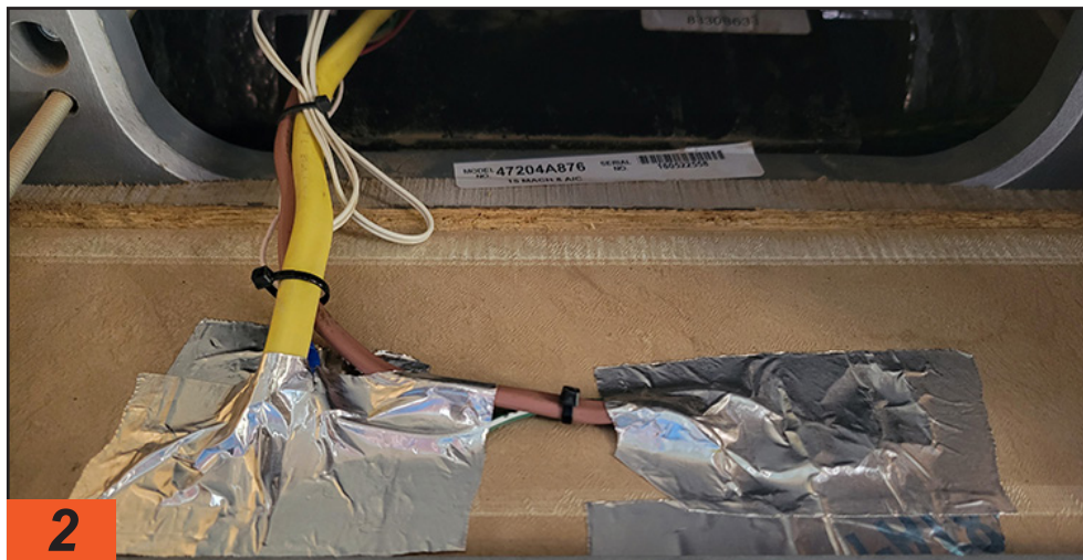
2 While sealing the holes in the return-air duct, time also was devoted to cleaning up the wiring. Cable ties were used to bundle the wires. This made working in the area much more palatable.
