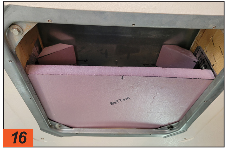
16 Before taping the wedges into place permanently, make sure the bottom plate fits properly in relation to the two upper wedges.
