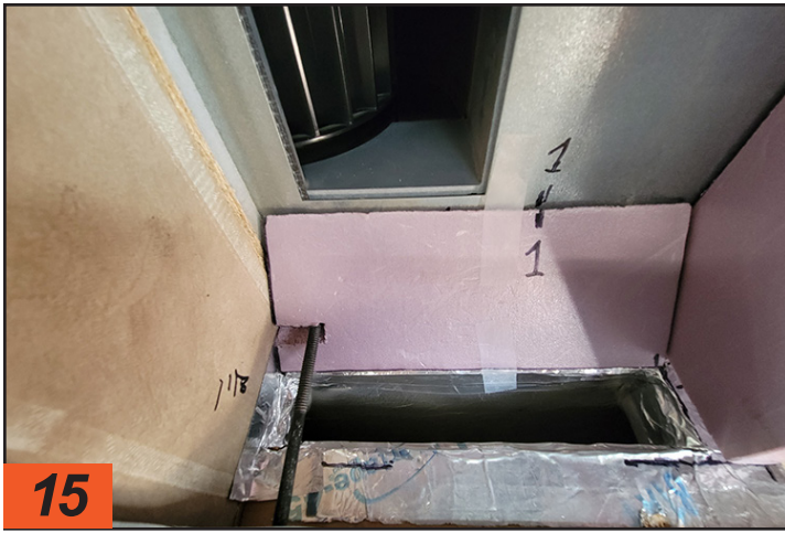
15 With one of the wedges taped into place, the vertical plate is positioned to make sure it is at the edge of the air duct.
