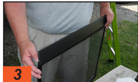
3 The extrusion was fitted to the bottom of the metal mesh screen protector before placing it in the screen channel.
