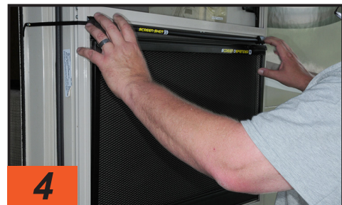
4 Once the Screen Defender is in position, the spring-loaded latches are employed, locking the metal mesh in place.
