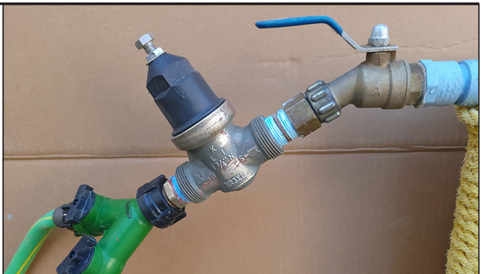
The Zurn Wilkins regulator is half the price of the Watts unit and has held up nicely over the last five years even though the top portion is made of a hard plastic material versus brass on the Watts model.
