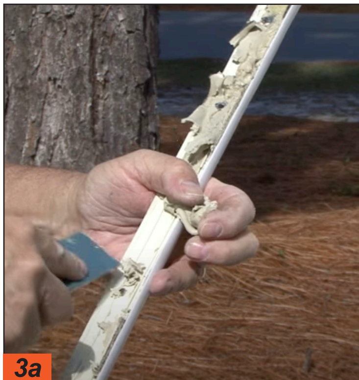
1 To begin, remove the molding insert to reveal the screws affixing the molding to the corner. If the old insert can't be cleaned, it can be replaced.
