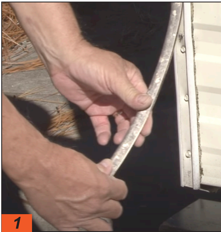
1 To begin, remove the molding insert to reveal the screws affixing the molding to the corner. If the old insert can't be cleaned, it can be replaced.
