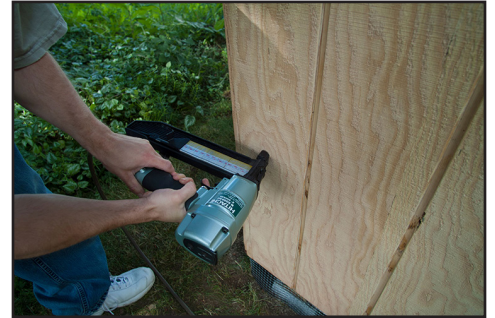
If wood is your choice for skirting your fifth wheel, T1-11 is the best product as it's designed for outdoor use. Just make sure the bottoms of the panels don't contact the ground. You'll need to find some way to block the air flow between the ground and the T1-11.
