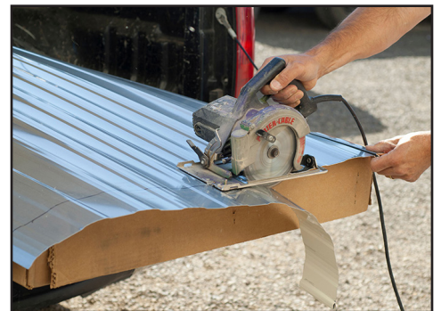
Fiberglass and aluminum designed for RV siding is also a good alternative to vinyl or fabric skirting if you aren't planning on moving your trailer for a long time. Installation requires some form of framework to hold it in place like T1-11 and other hard panels used in skirting a trailer. (Photo by Larry Walton)
