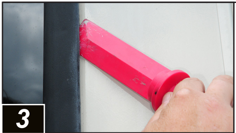
Since the window on the project fifth wheel was replaced a few years back with an aftermarket version, the outer frame continued to stick to the door panel. A plastic pry bar was used to release the frame from the butyl tape.
