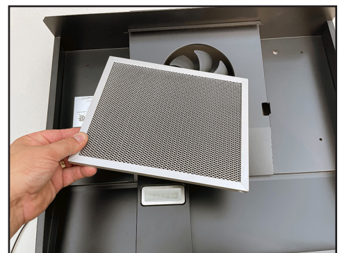
The range hood needs service, as well. Keep the filter(s) clean and check to make sure there are no nests in the hood or duct. RVE
