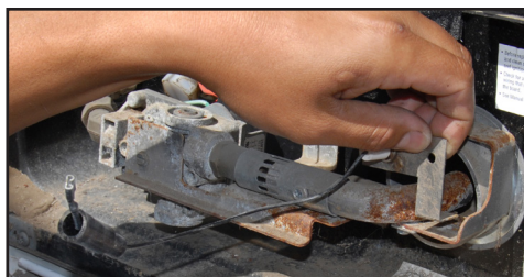
With the screw removed, the ignitor bracket assembly can be lifted out of the way.
