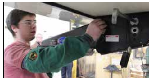
Using a drift/centering pin (or screwdriver), center the holes and install at least one bolt on each side in different locations to support the weight of the new pin box for final assembly.
