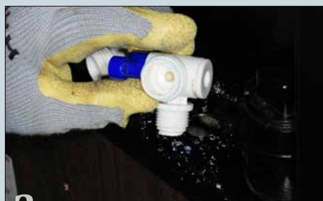
2 Stock, plastic faucets were cut off using a hack saw blade. There was not enough slack in the Pex tubing to pull up through the mounting plate in the wall to cut off the faucet below the hose clamp. Once separated from the hose, the plastic faucet was discarded.
