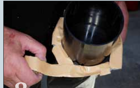
8 Butyl tape, provided with the kit, was placed around the flange that rests against the surface of outside wall.
