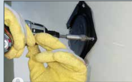
9 The vent tube fit perfectly. To prevent moisture intrusion self-drilling screws were coated with a silicone sealant before securing the flange of the vent tube against the outside wall.
