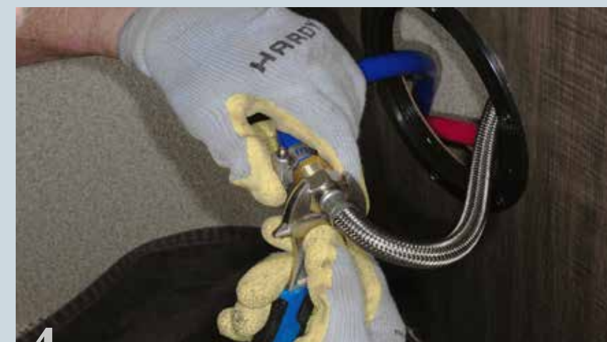
4 A brass, barbed fitting was installed in the end of each Pex tubing. This fitting allows attachment of the new faucets (turn-off valves). Adding stainless steel hoses made it easy to attach the new faucets and mount them back in the original housing in the wall. Replacing the faucets is not mandatory, but the added reliability of the brass fixtures, and the fact that they could not be opened and closed once the washer and dryer were in place, instilled greater confidence for the owner of the fifth wheel.
