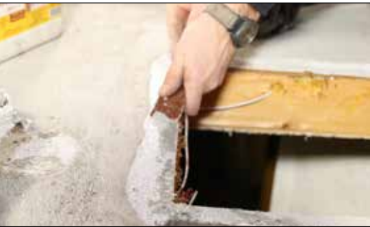
Up on the roof, carefully remove the sealant around the existing fan. Using heat may help but be very careful not to damage the roof membrane or surface. Remove all the screws and peel up the fan. Once up, again try to remove as much of the old sealant as you can without damaging the roof.
