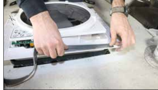
Apply sealant tape to the flange around the inverted fan. The technician at Tim's RV used double-sided EternaBond tape, but regular butyl tape will work also. Make sure the tape goes all the way around.
